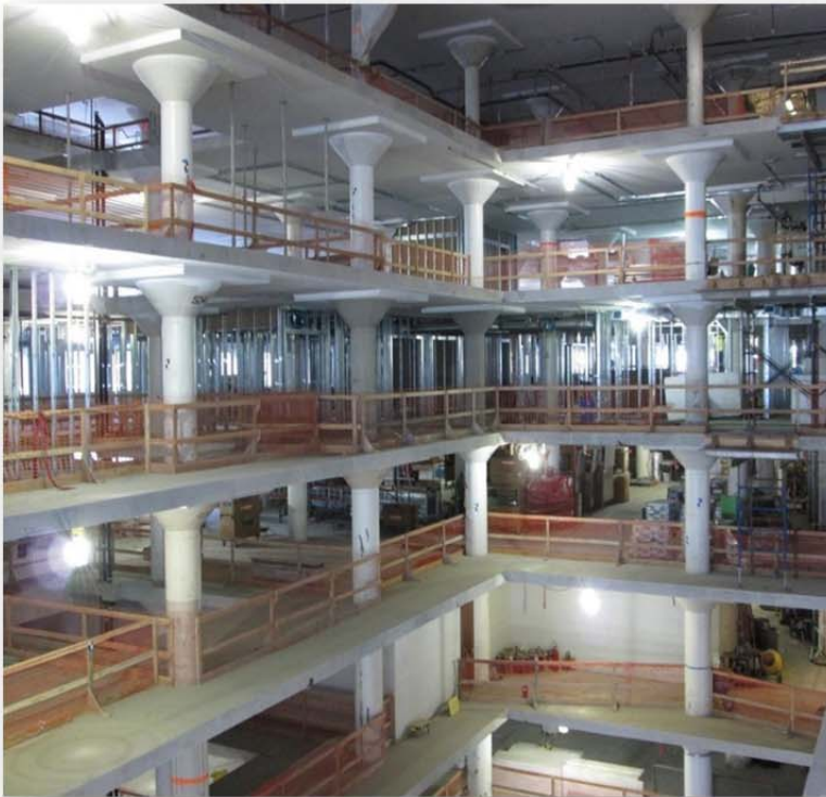
Figure 1: On Level 6, installation of framing, utilities and plumbing overhead.
