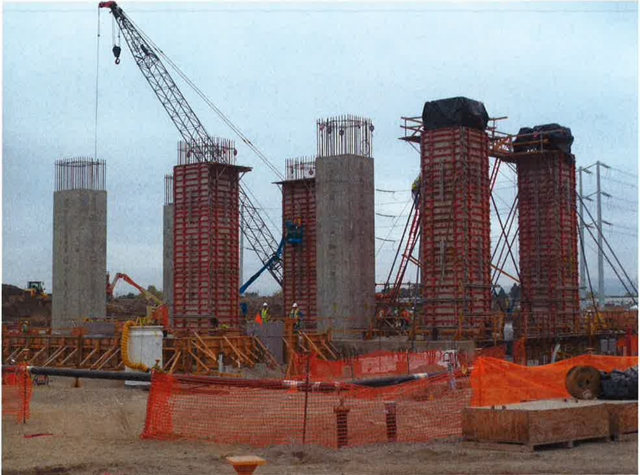
Photograph #2 Pillars for elevated installation of the steam turbine
