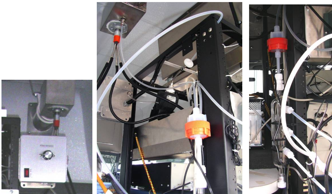
Photos of the inlet duct and fan control, stainless steel plenum exiting duct, and glass plenum with particle filter (replaceable paper disk filter is in the orange cartridge).
