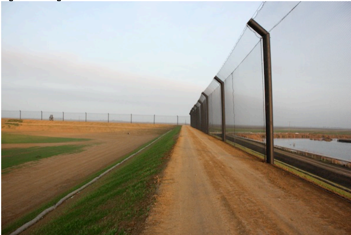
Figure II-7: Fugitive Dust Control with Wind Screen
