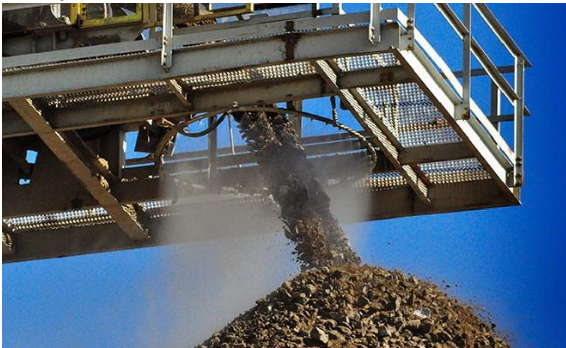
Figure II-5: Spray water fog and mist to keep disturbed surfaces damp during bulk material moving operations.
