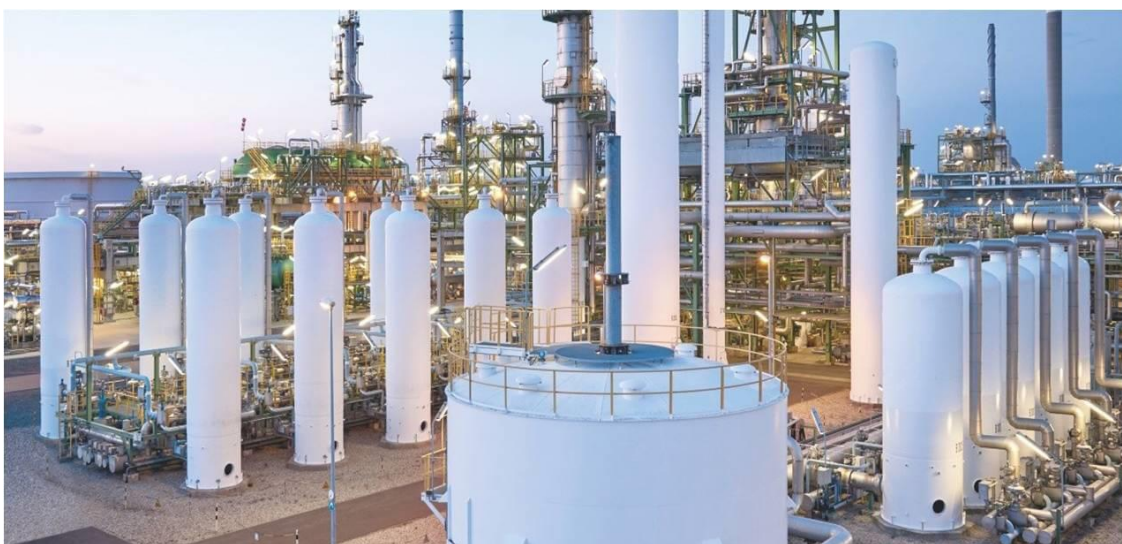
Figure 6: Image of several tanks containing the adsorbent material that comprise part of a pressure swing adsorption system
