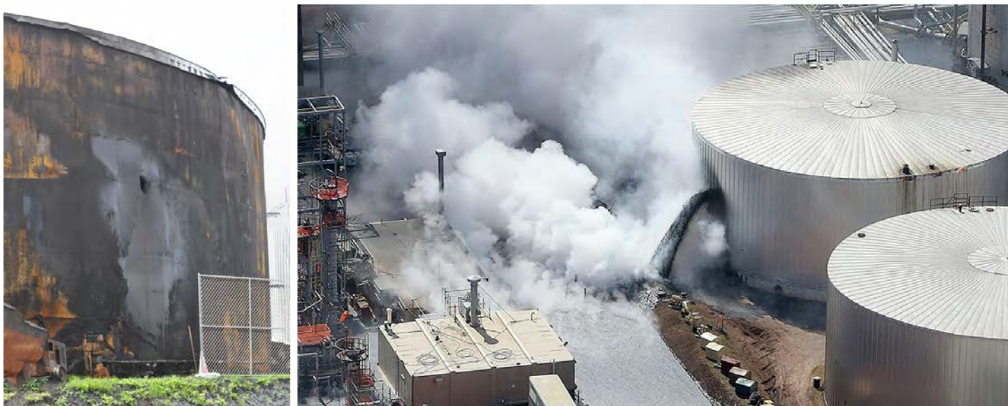
Figure 4. Post-incident photographs of the leaking Asphalt Storage Tank. Debris from the explosion punctured the side wall of the tank creating a large asphalt leak outside of the secondary containment area. Credit: CSB (left) Duluth News Tribune (right).
