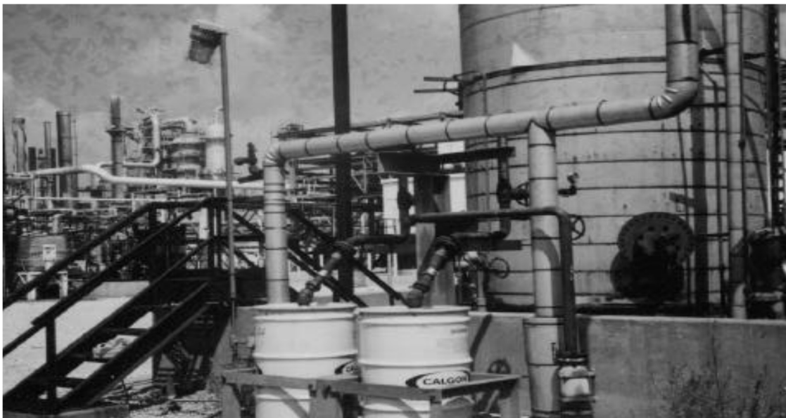
Figure 4 Use of Carbon Adsorption for Control of Wastewater Collection Systems at a Refinery
