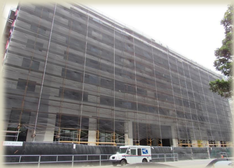
Exterior scaffolding for exterior painting
