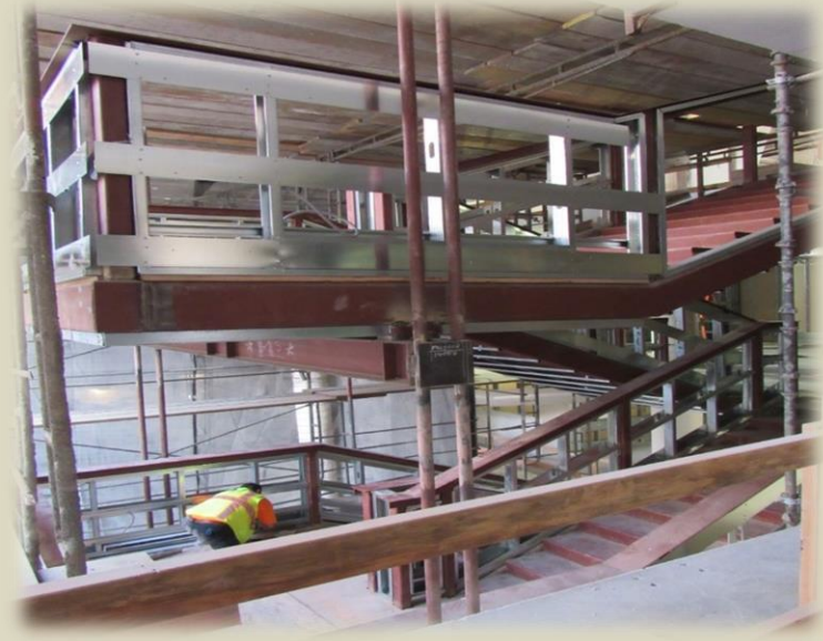
Steel enclosure for hanging stair case
