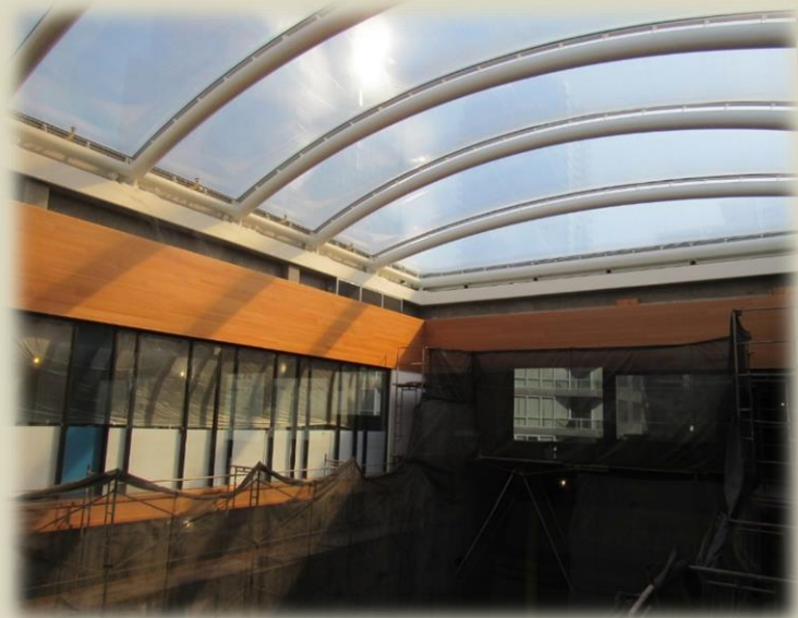
View of atrium skylight with wood and glass framing
