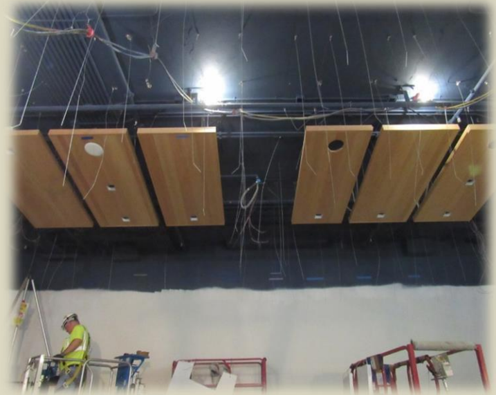
Wood ceiling finishes and acoustics underway
