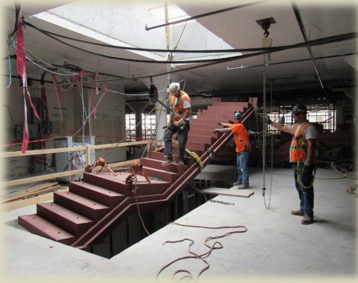
Installation of hanging stair case
