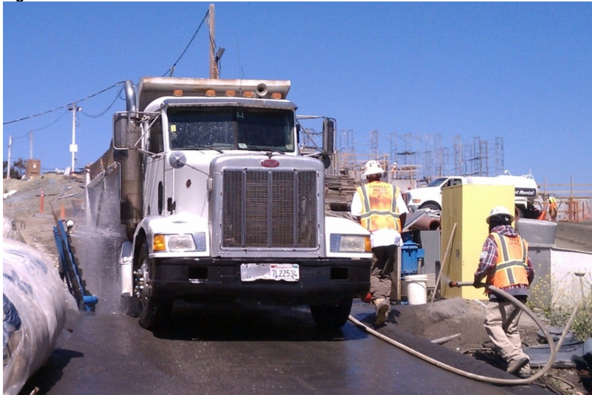
Figure II-4: Truck-wash Station used to control Trackout
