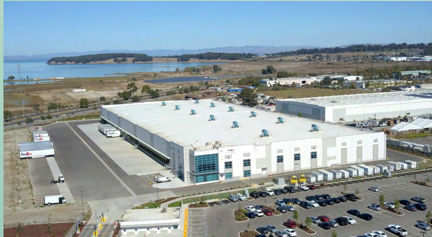
FedEx ZEV facility in North Richmond. Source: Overaa Construction
