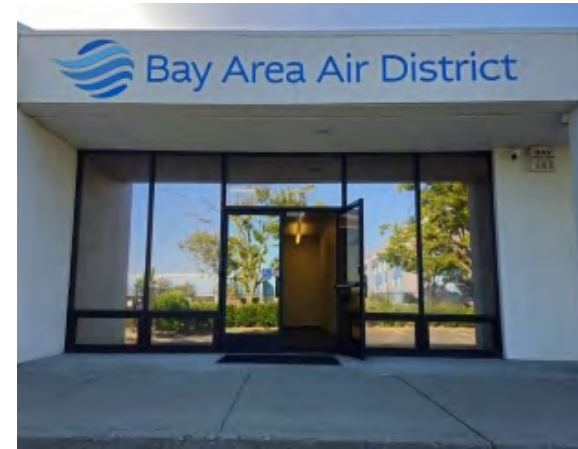
Headquarters East (HQE) 4114 Lakeside Drive, Richmond
