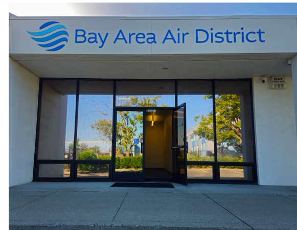
Headquarters East (HQE) 4114 Lakeside Drive, Richmond
