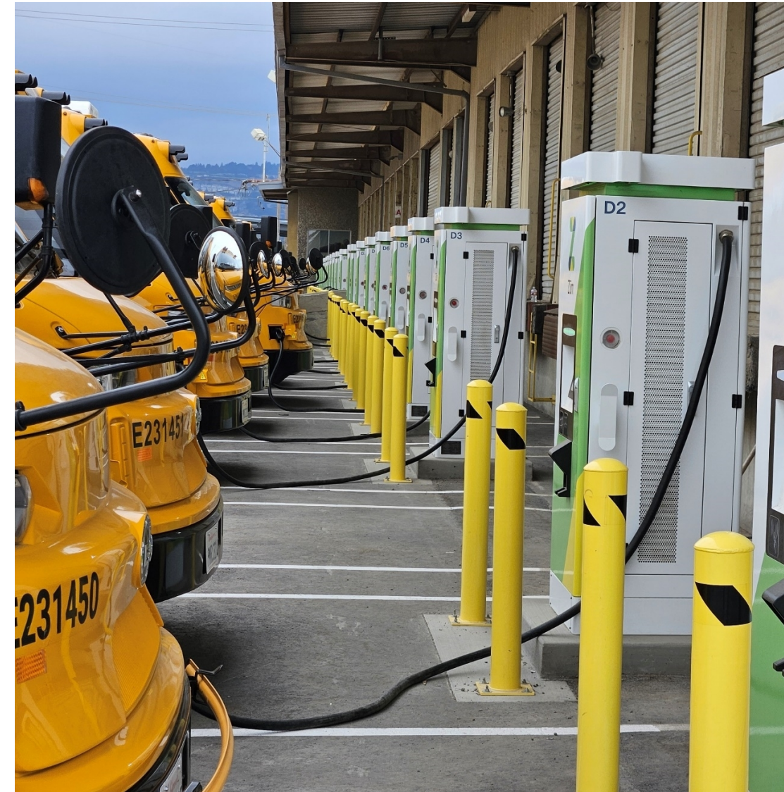
Source: Air District equipment inspection
