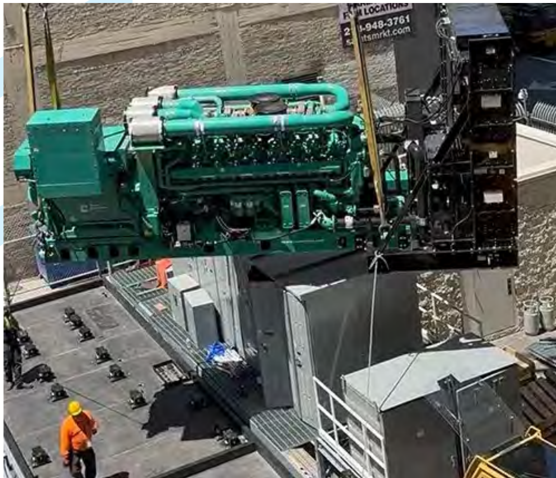
Diesel Generator at a Data Center in Los Angeles (Creative Commons)
