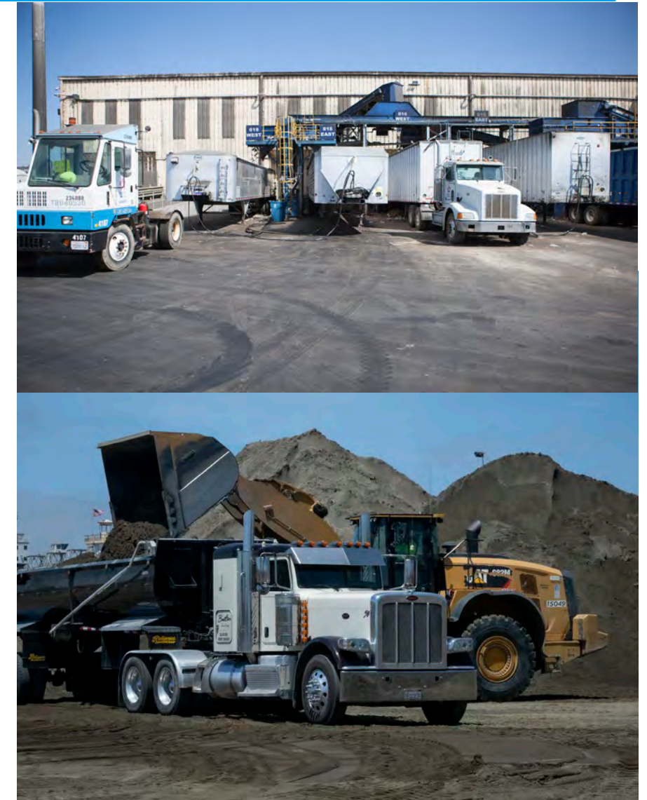
A material handling facility and a construction site.
