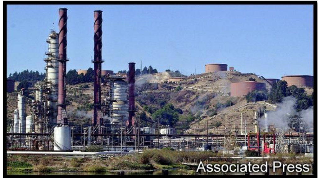
Chevron oil refinery, Richmond, CA ( www.wtsp.com )
