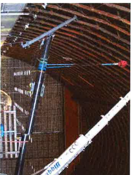
Hoisting of temporary shore segment
