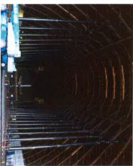
Temporary shores after installation
