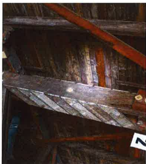
Typical chord member with battens
