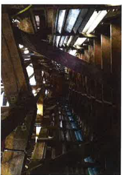
Roof monitor deflection in critical zone
