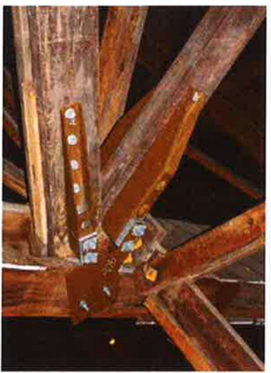
Typical connection strengthening bracket
