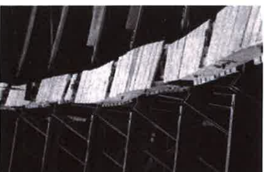
Buckled chords (left) and glulam strongback repairs (right) - "Restoration of Navy LTA (Lighter than air) Hangars", Donal Neal, 1986
