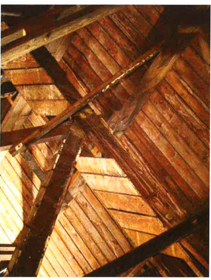
Typical vertical web member with added knee-braces
