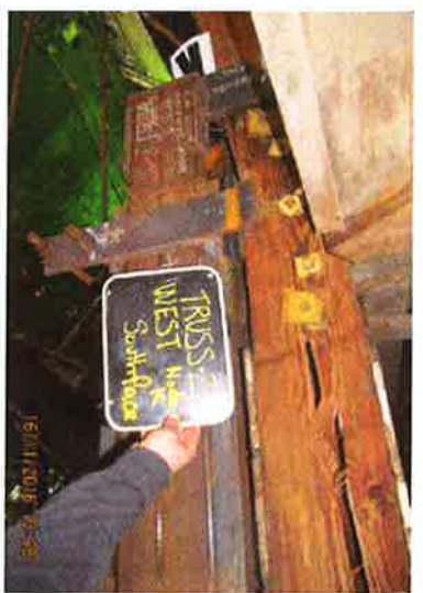
Chord damage at node K after exoskeleton install
