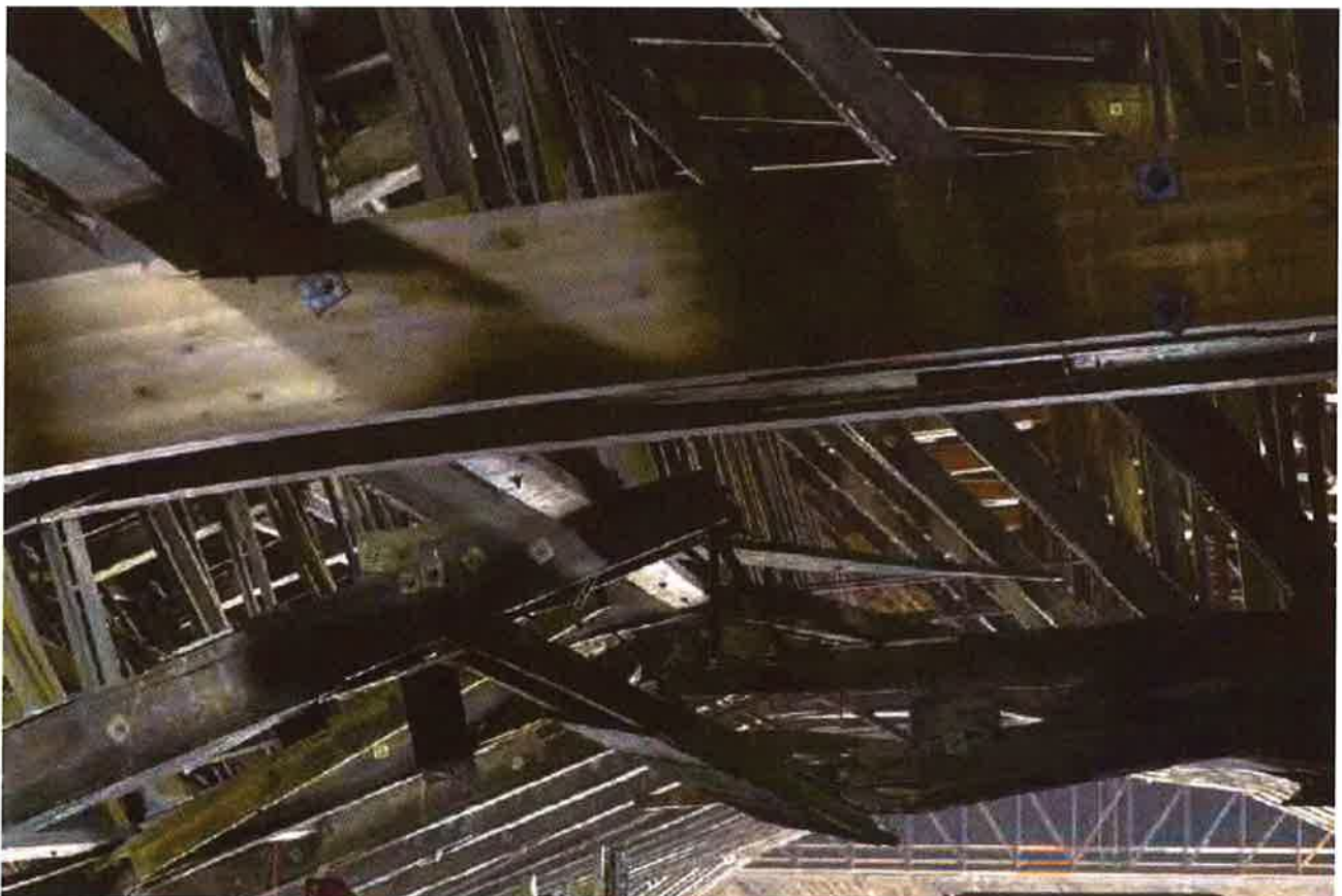
Figure 6. Broken bottom chord near top of truss.
