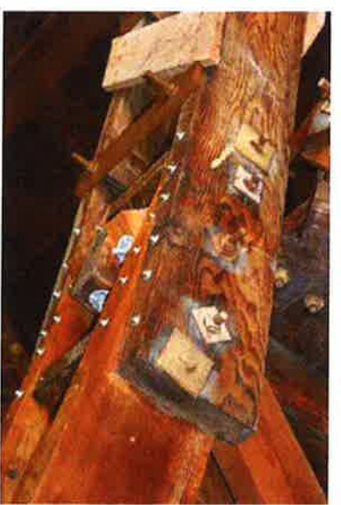
Preemptive screw and clamp strengthening on undamaged chord at node K
