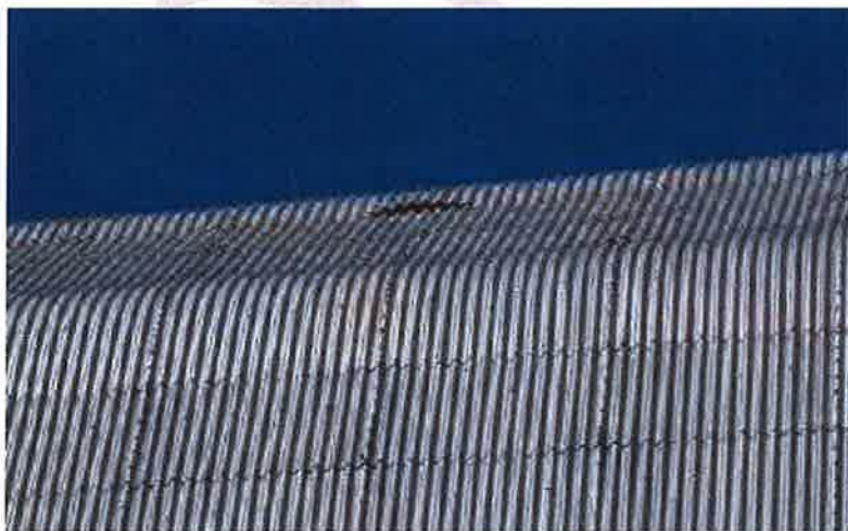
Figure 10. Example location of detached corrugated aluminum sheathing on roof exterior of Hangar 2.
