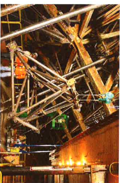
Hoisting exoskeleton segment into place
