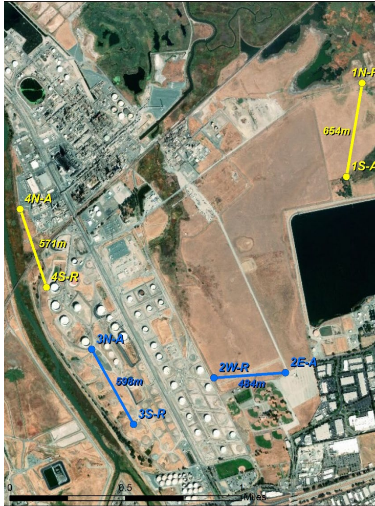
Figure 2. Open-path monitoring sites for the Martinez Facility. The four paths are labeled 1N-1S, 2E-2W, 3N-3S, and 4N-4S, with 'A' and 'R' denoting whether the site is the location of an analyzer or reflector, respectively.
