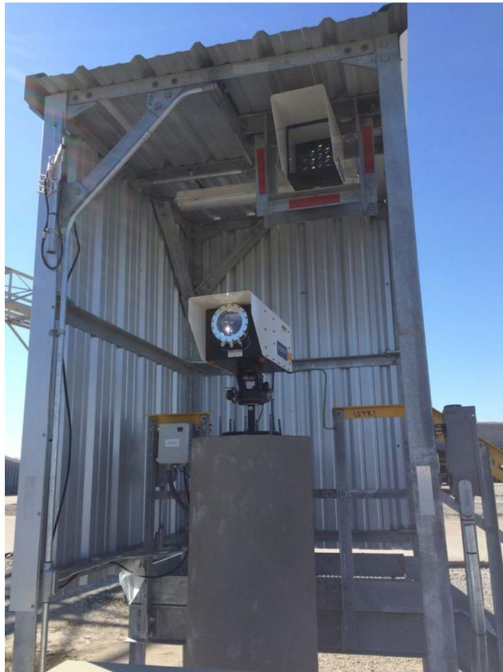
**Figure 17.** Example of a UV-DOAS analyzer installation.
